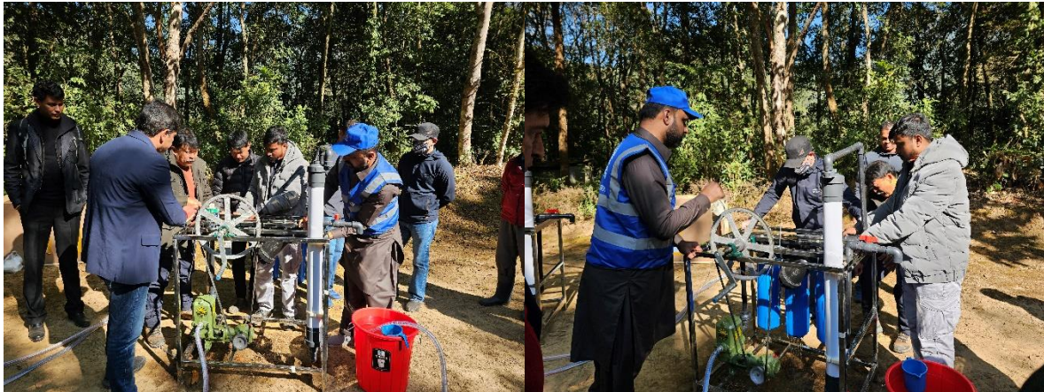
Assembly and testing of filtering unit
